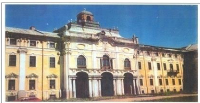
Figure 22: View from the Southern Facade of Konstantinovsky (19)
