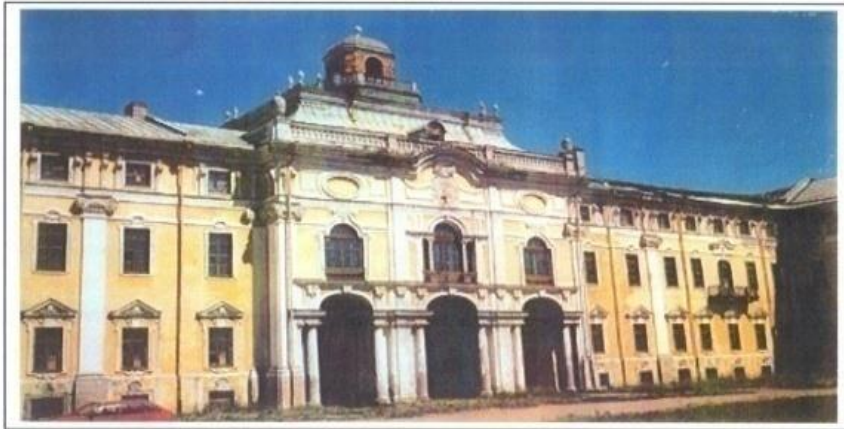
Figure 22: View from the Southern Facade of Konstantinovsky (11)
